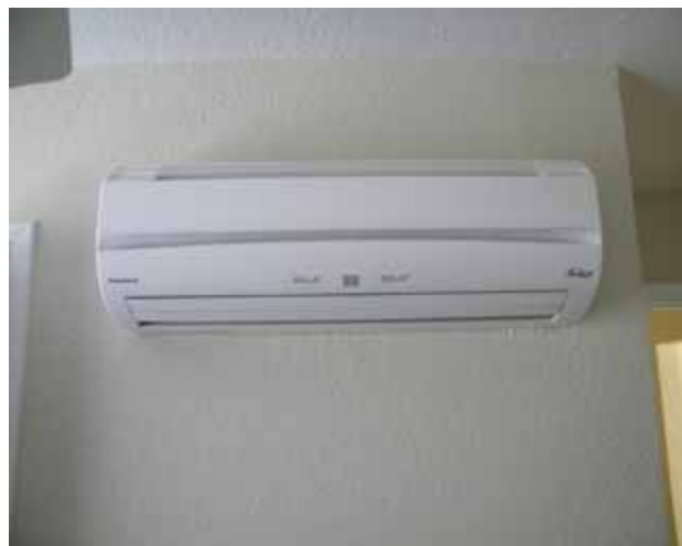
Mini-Split Indoor Air Handler
